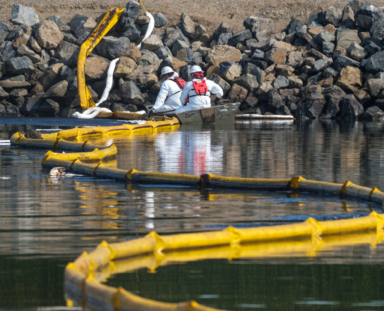
Crews deploy skimmers and floating barriers known as booms to try to stop further incursion into the Wetlands Talbert Marsh in Huntington Beach on Oct. 3, 2021. AP Photo/Ringo H.W. Chiu
